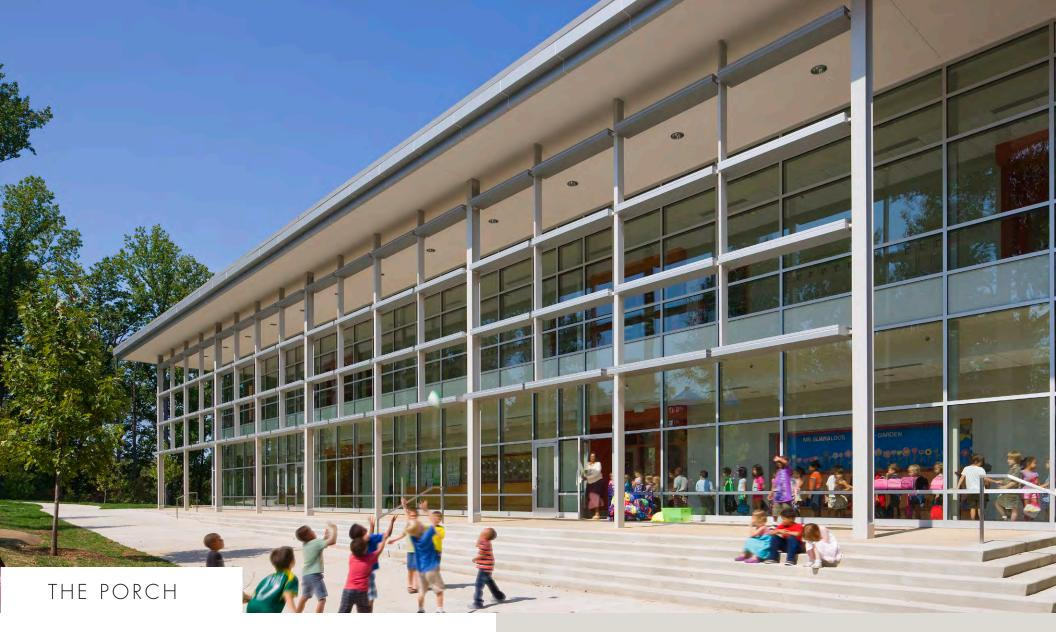
This loggia, called "the Porch", creates a transitional environment between indoors and out and is designed to shade the addition's south facing curtainwall in the peak cooling months. During the winter the sun enters the building to warm the terrazzo floors inside the curtainwall helping to passively heat the building.
