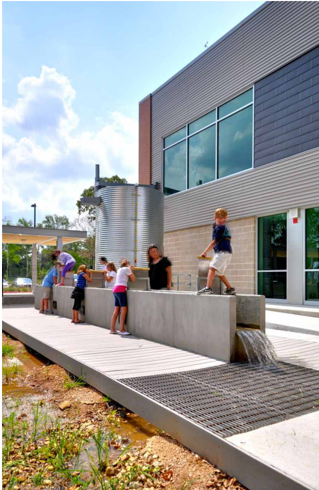
Water collection cistern/Erosion trough.
