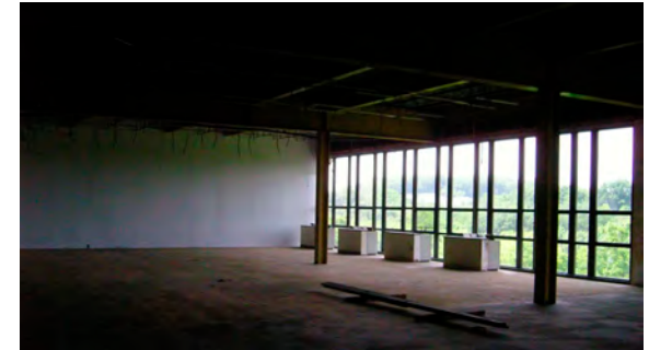
Library Space Stripped to Structure (2008)
