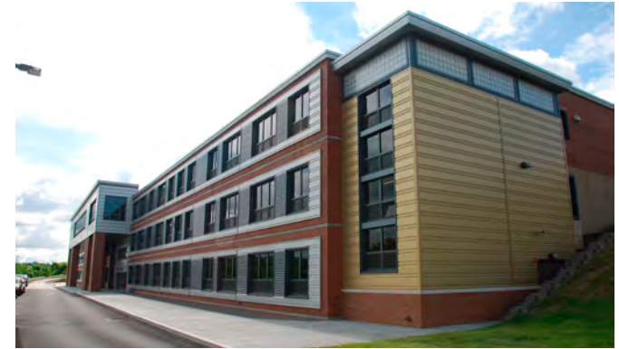
STEM Building After Renovation
