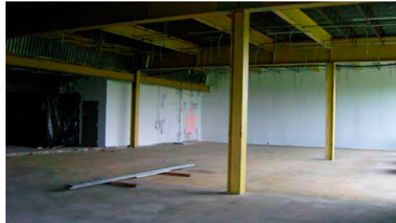
Library Space Stripped to Structure (2008)
