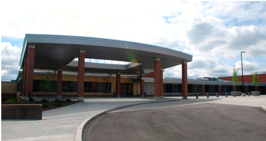
High School Main Entrance Canopy
