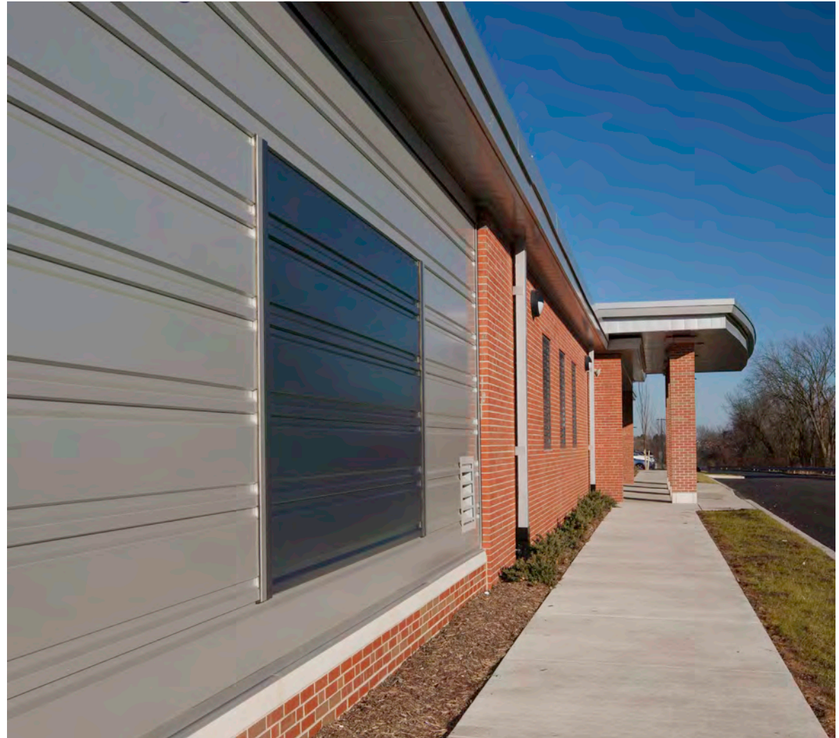
Intermediate Gymnasium Exterior - Metal and Brick interface where New Addition Meets Renovated Building
