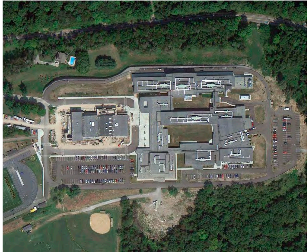
Aerial Photograph of Campus Site, During Construction of the Athletic Center
