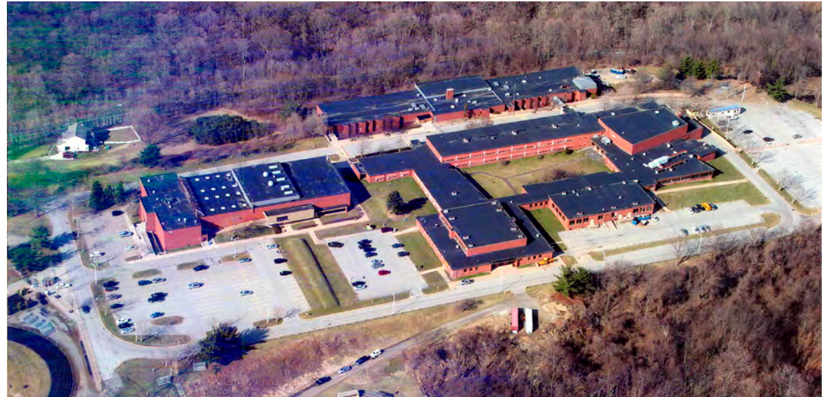
Aerial Photo of Campus Prior to Renovations
