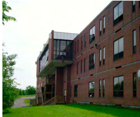
STEM Building Prior to Renovation
