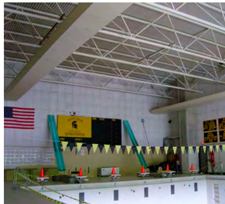
Natatorium Prior to Renovation
