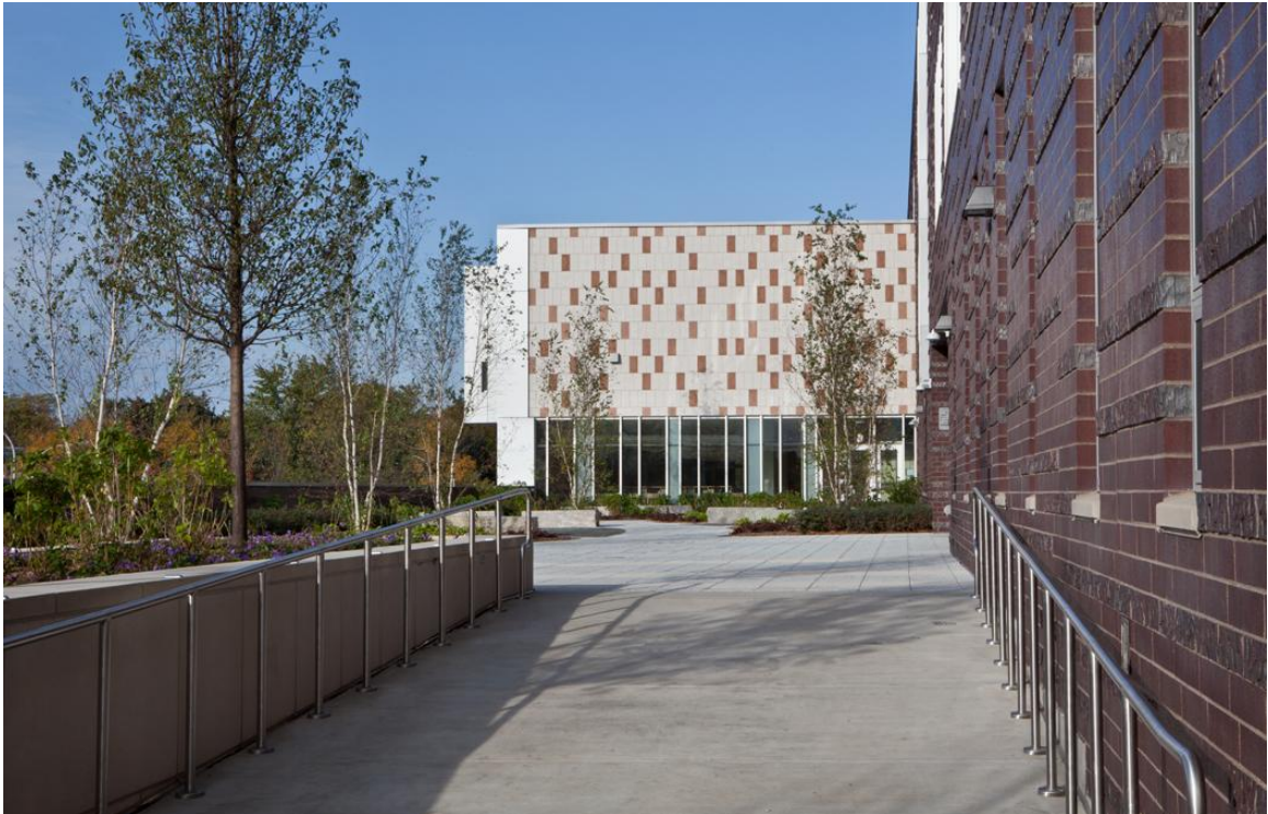
Reading garden with entrance to the library
