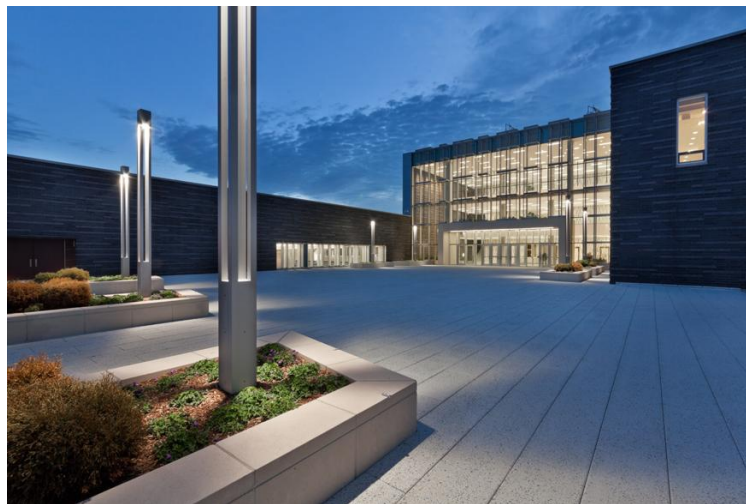
Efficient lighting systems
