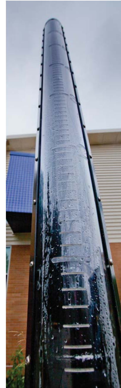
▲ Rainwater cistern gauge
