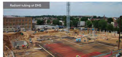
Radiant tubing at DHS
