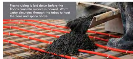
Radiant tubing at DHS
