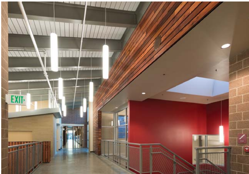
Exposed tubular daylighting devices transmit daylight to the interior levels of the building.
