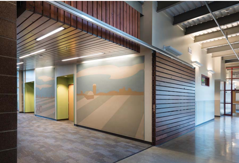
Reclaimed lumber and decking from the demolished Anna Bryce School in multiple locations express the heritage of the community and demonstrate the ability of new buildings to reuse existing materials.
