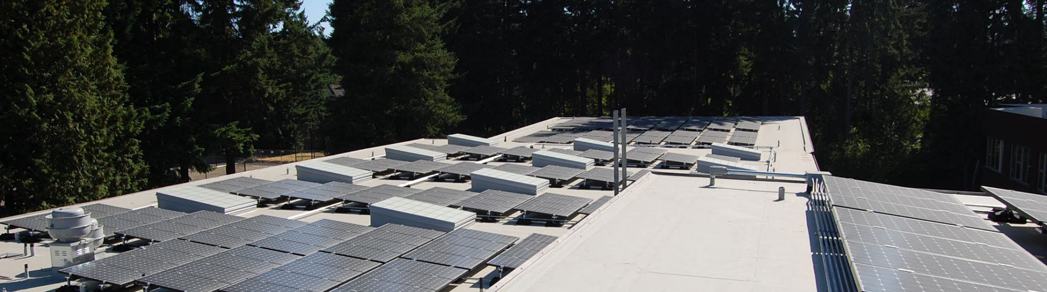
100 kW photovoltaic array produces energy that often goes back to the grid.
