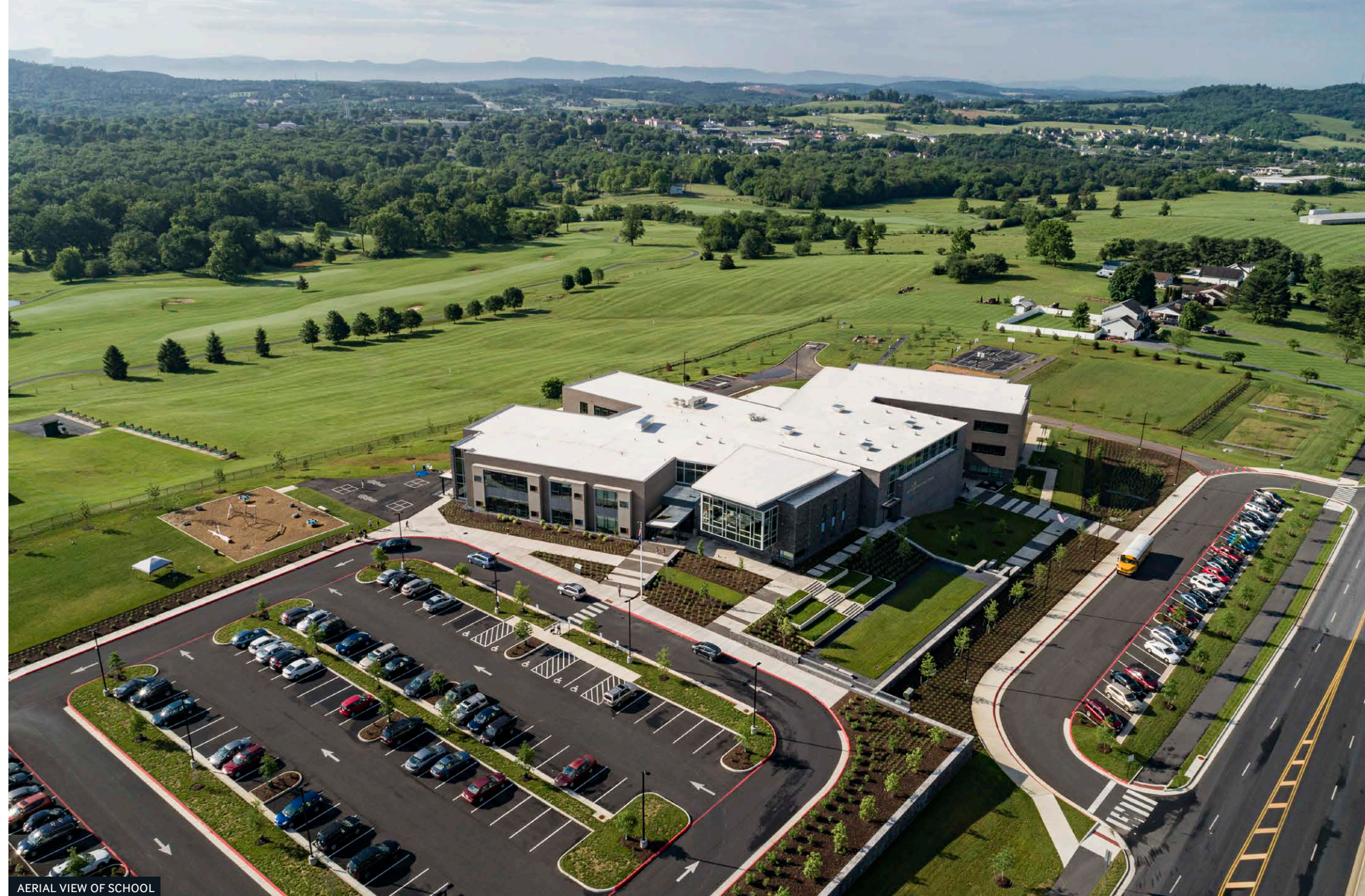
AERIAL VIEW OF SCHOOL
