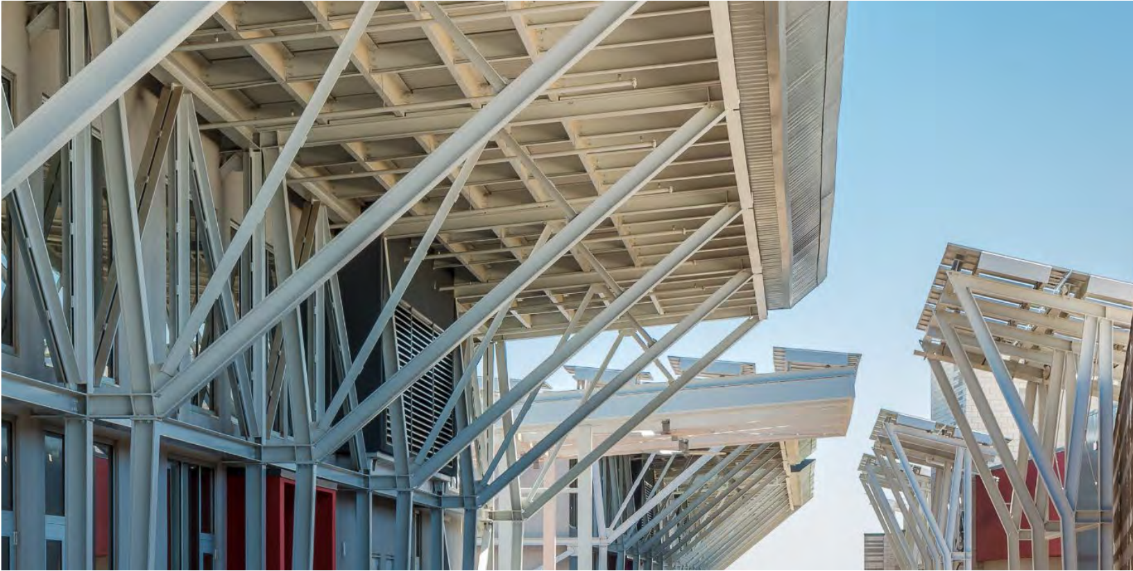
An open roof structure with solar panels allows night heat to re-radiation to the atmosphere.
