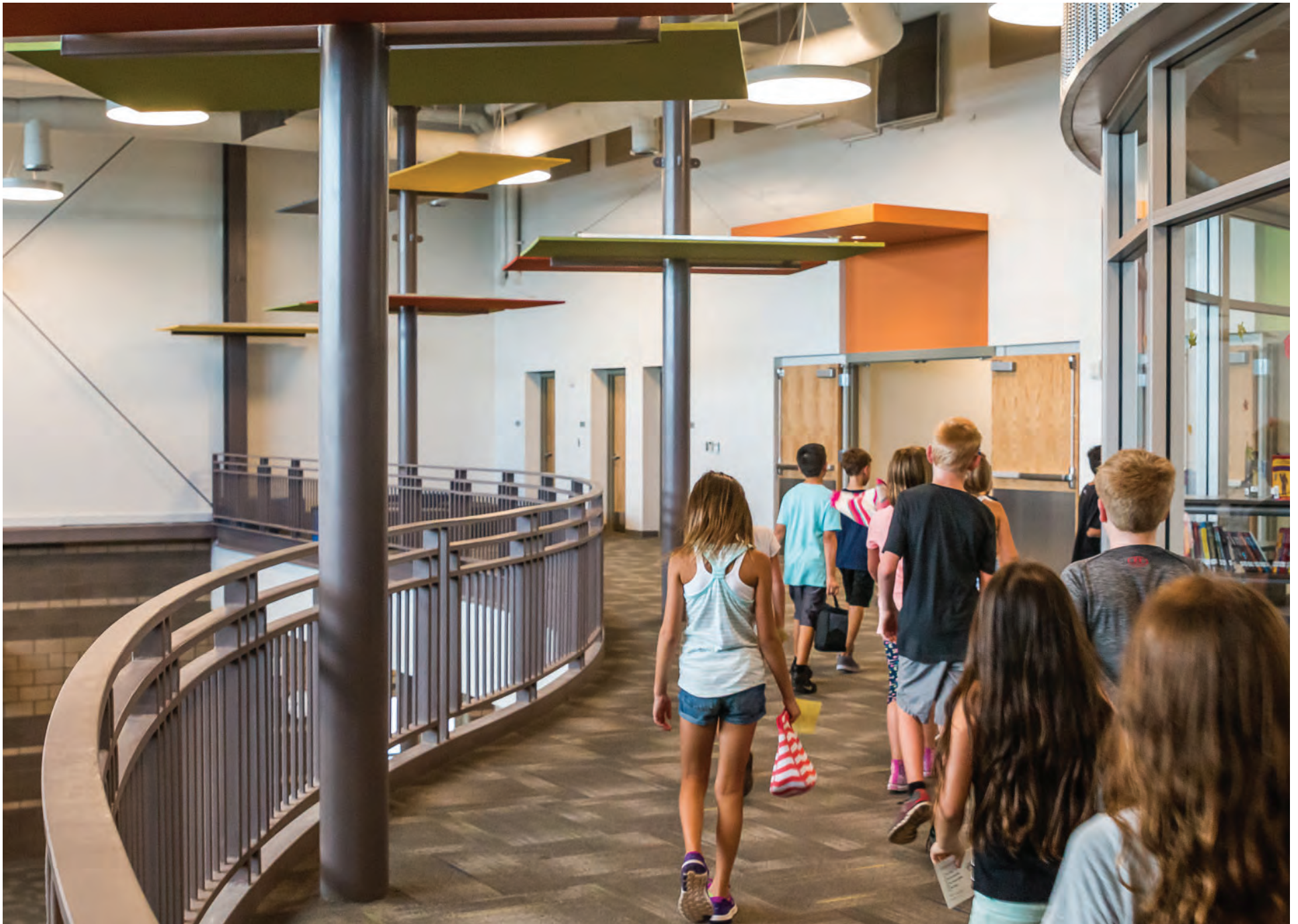
Acoustic “trees” support the balcony and, along with the perforated metal sound soak panels above the Media Hub, help to control noise in the Commons.
