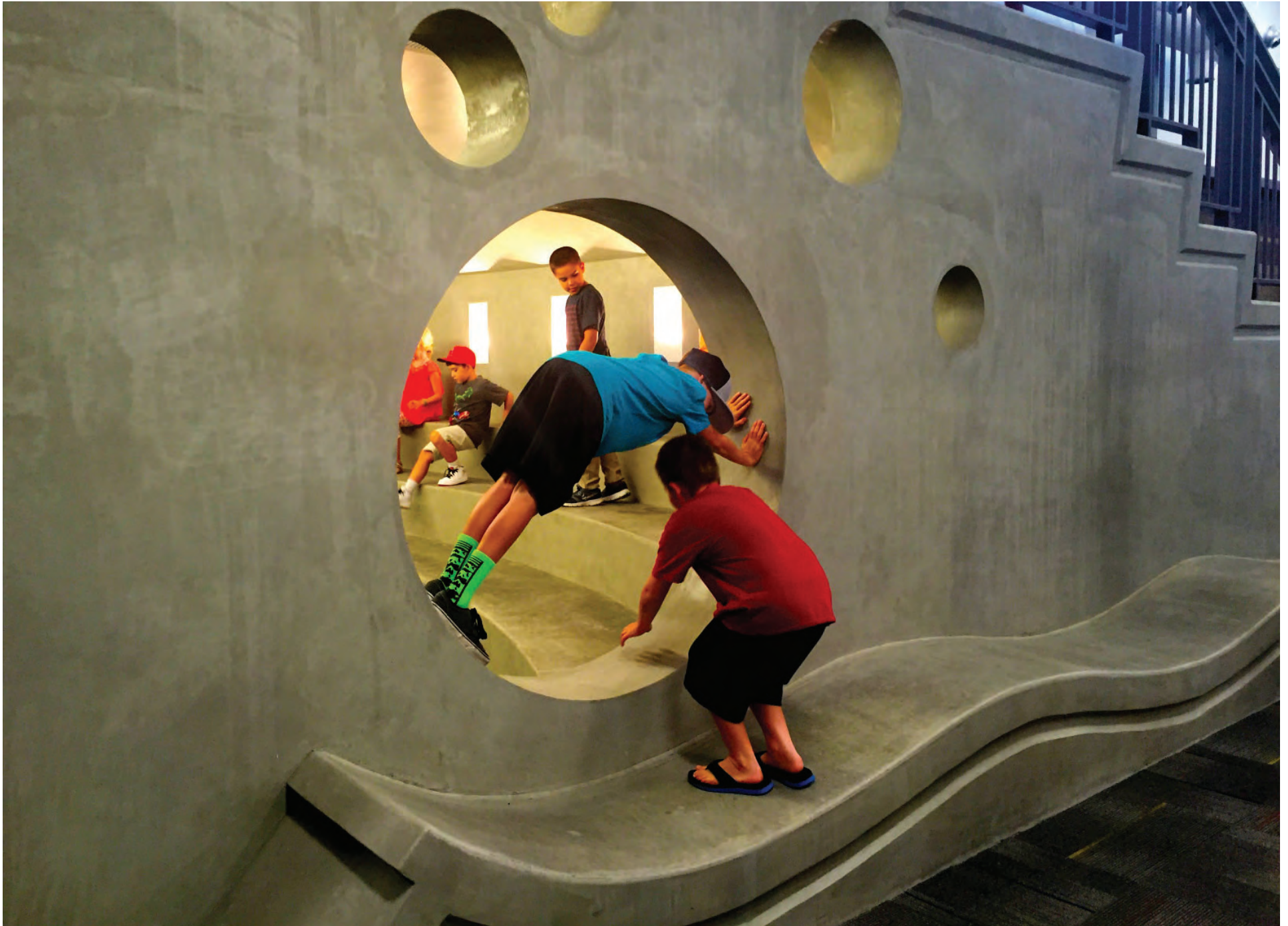
The “Troll’s Lair” reading / storytelling nook design under the stairs takes advantage of the properties of cast-in-place concrete.
