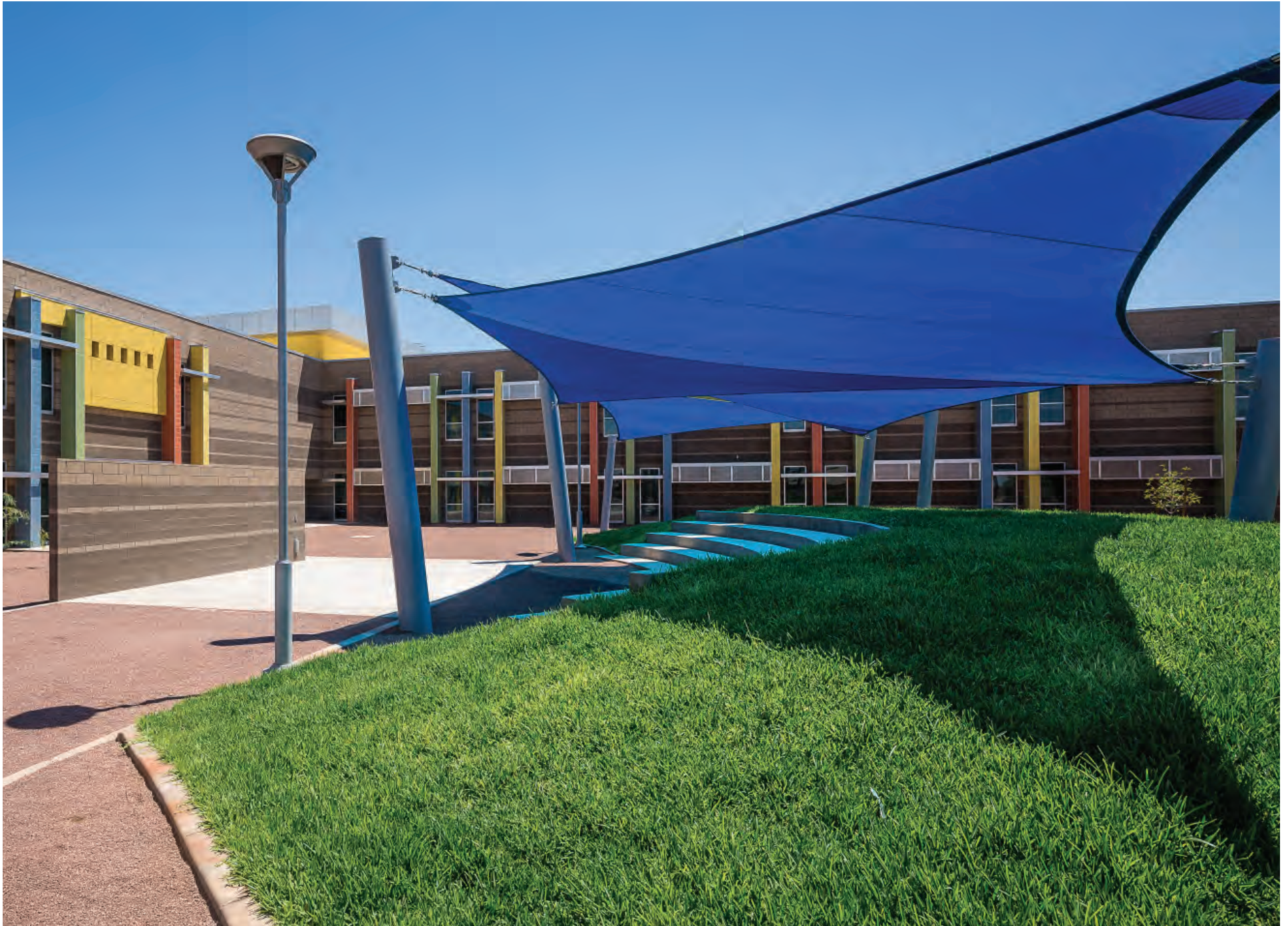
Tensile structures, creative and cost effective, provide much needed shade all around the site, including over the amphitheater on the southwest side.
