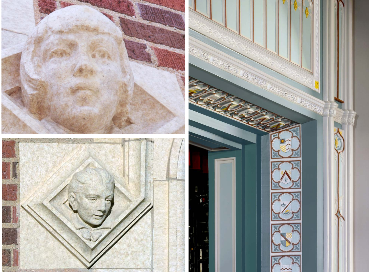
Restored exterior terra cotta and interior decorative plaster.
