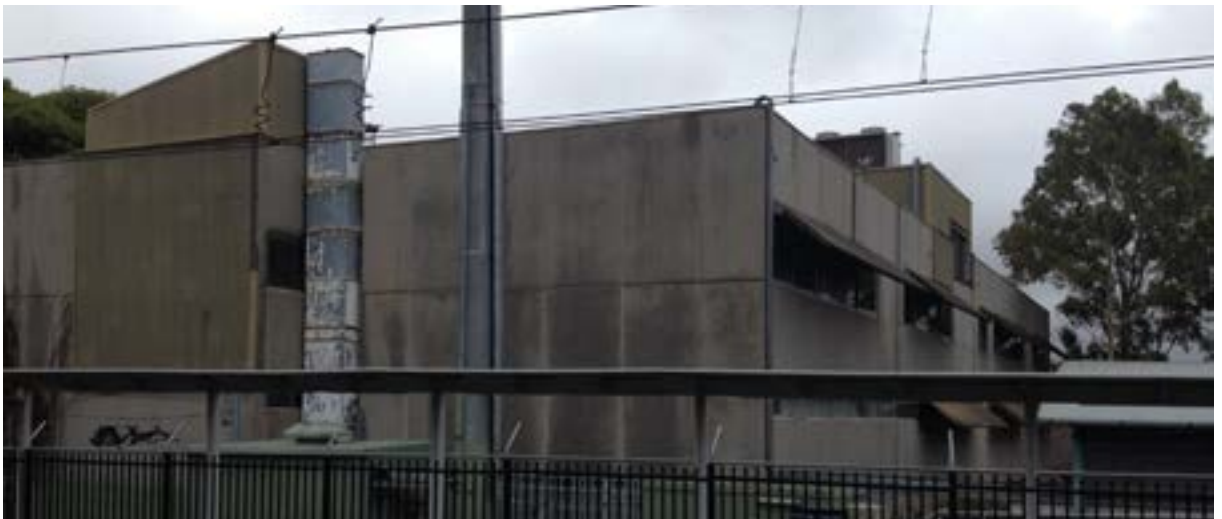
The former Telstra training centre before the renovations and additions in Stages 1 and 2 of the project
