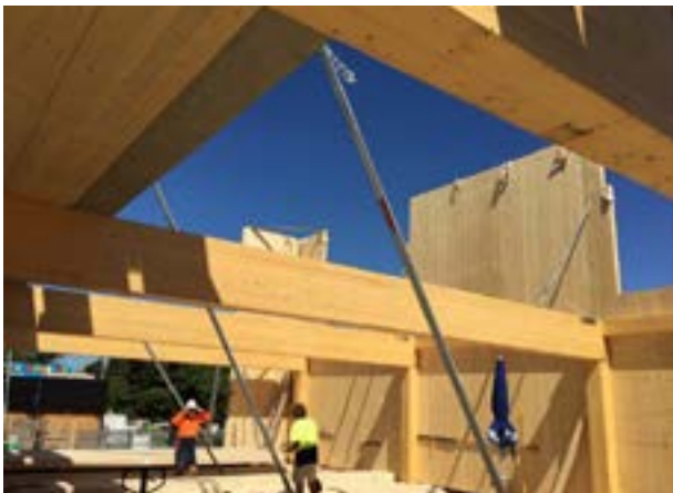
Installation of Glulam and CLT walls and acoustic ceiling flooring systems
