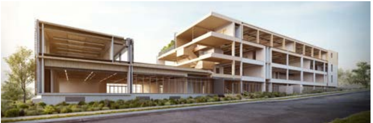
Cutaway showing timber structure
