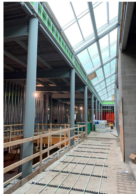
Skylight and radiant floor heating under construction
