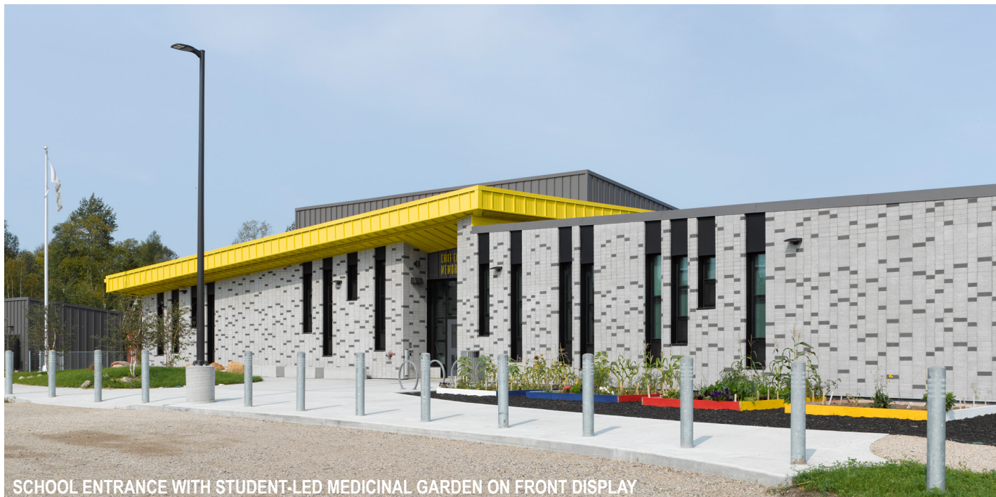
RAKED VERTICAL MORTAR JOINTS FLUSH HORIZONTAL MORTAR JOINTS
