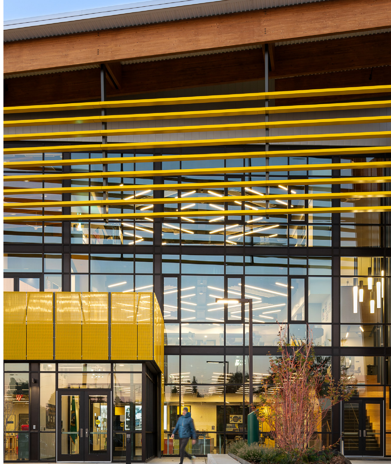
A simple shed roof spans the double height volume, supported on heavy timbers which reflect an association with the Pacific Northwest region.
