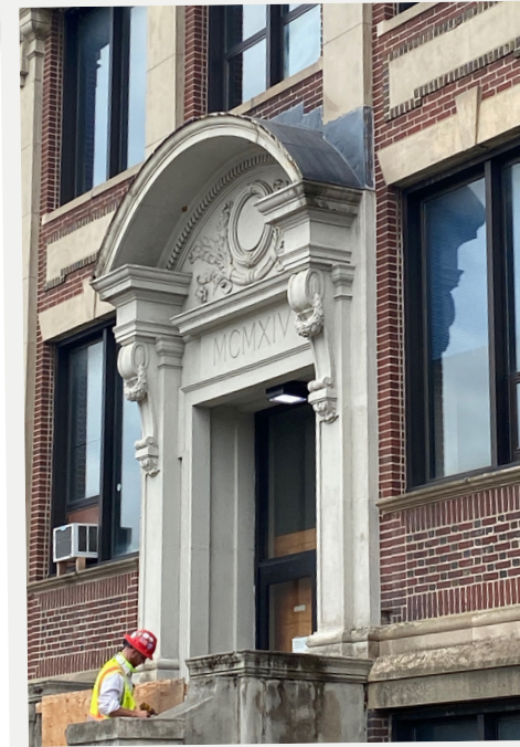
The stone facade of the original 1914 AHS Fusco Building was preserved, restored, and now serves as the entrance to the black box theater, connecting generations of students to Arlington's history.
