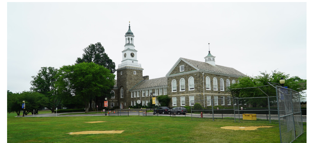
The original 1925 campus buildings show Colonial Revival architecture with a distinctly simple Quaker interpretation.
