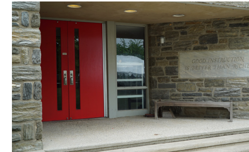
Existing lower school entrance.
