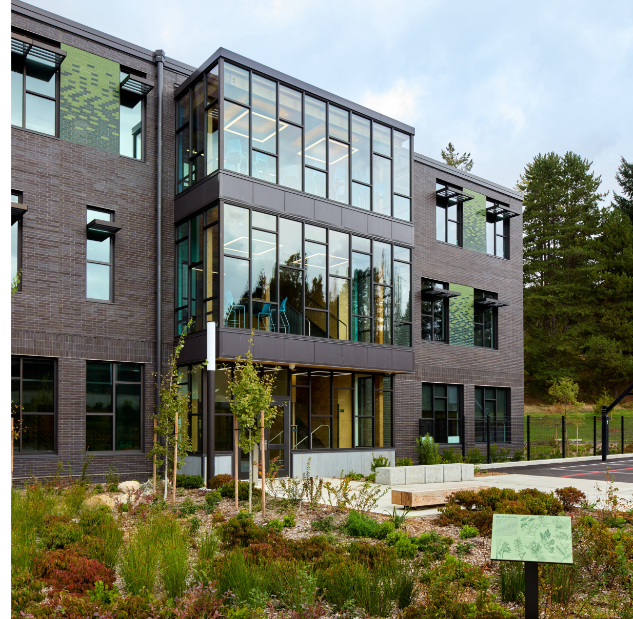
The exterior facade is a dark brick veneer pierced with glass “crystals” that highlight important gathering spaces in the school. The brick forms are accentuated by colorful glazed brick arranged in a blended pattern that seamlessly integrates with the surrounding landscapes.
