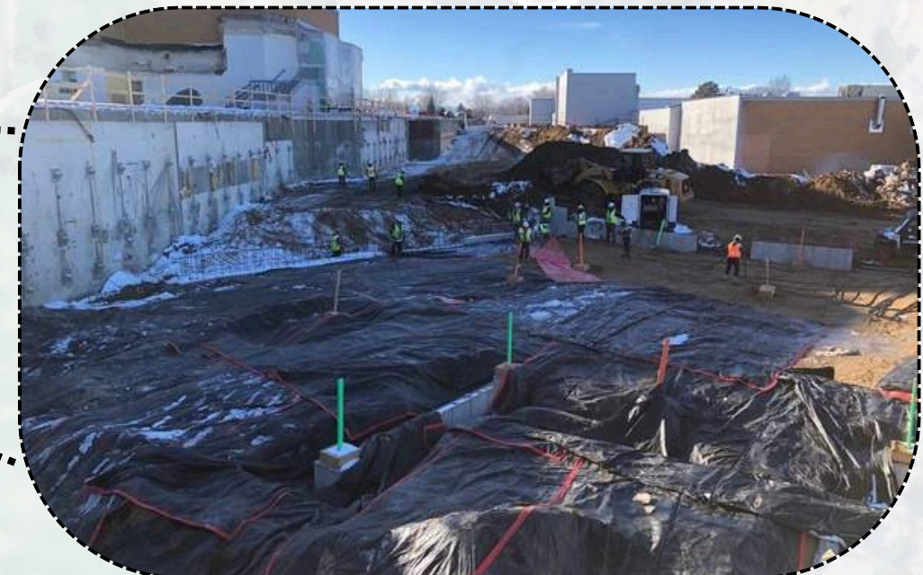
SHORING EXISTING BUILDING FOR USE IN NEW SCHOOL
