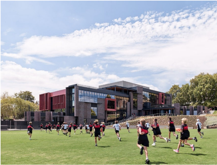
View from the Chapel Oval. Blue-brown brick forms erupt from the terrain, fragmented to create an inhabitable façade.
