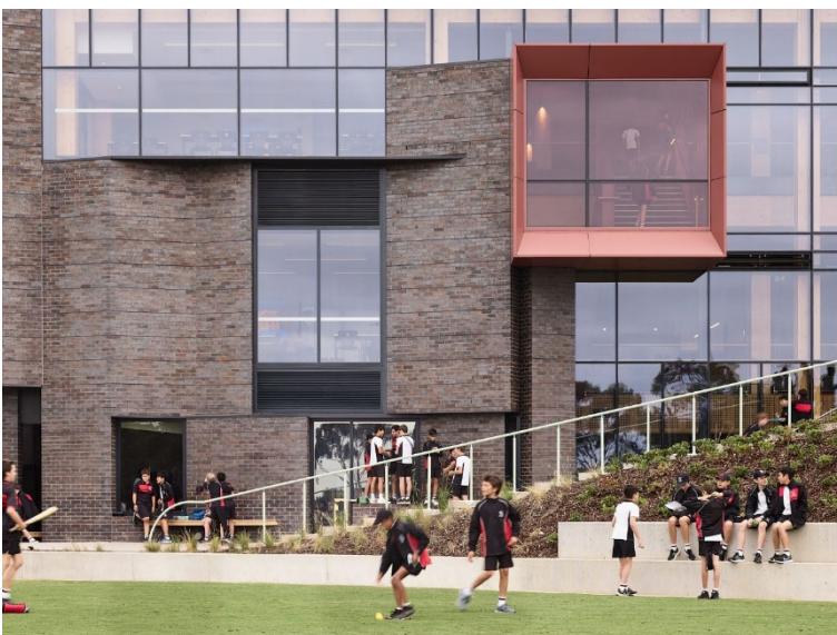
Southern elevation. Internal stairs connecting the leaning neighbourhoods are highlighted by red pop-outs on the external façade.
